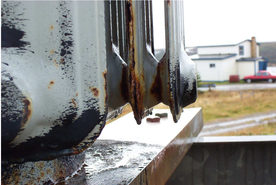
Pictures of Fall Pond transformer rusting
